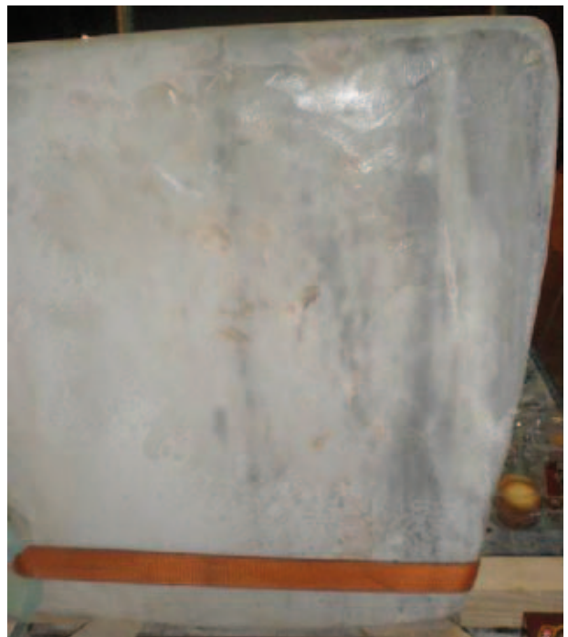
FIG. 5. Parallel grayish blue to gray bands visible in the transverse wall.
