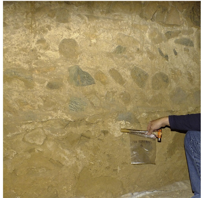
Fig. 4. Sample CanFer 006 was taken from stratigraphic unit 2032. Notice the stones in almost herringbone arrangement, a 4th, 5th and 6th century technique.
