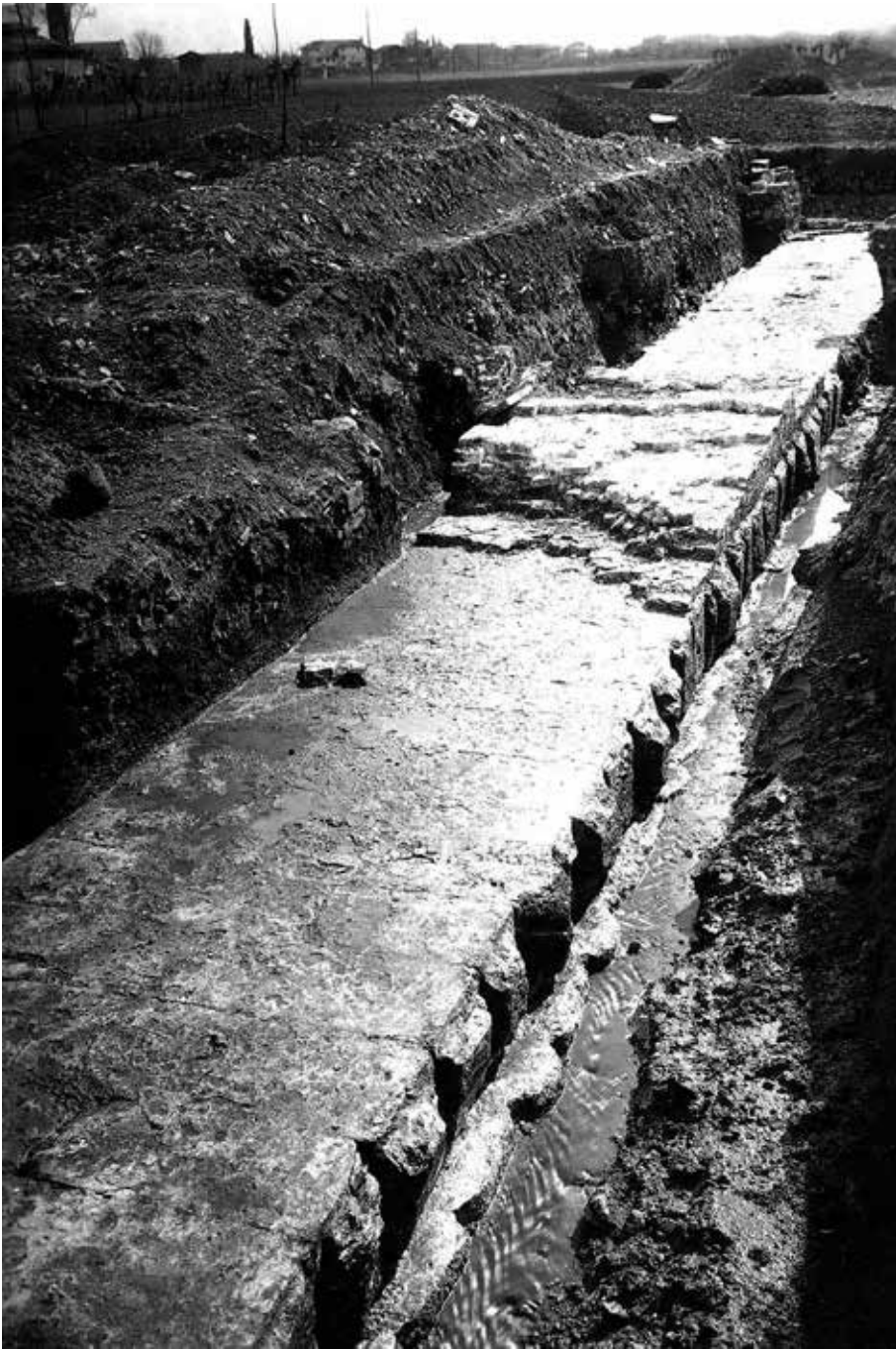
Figure 14.5: The western side of the republican walls of Aquileia. Foundations made of squared blocks of Istrian stone (Strazzulla 1989).
