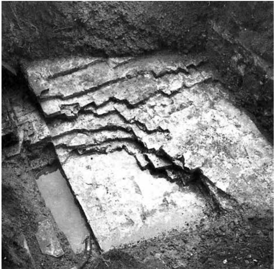
Figure 14.4: The republican fortifications of Aquileia: part of the wall made of fired bricks (Tiussi 2006).
