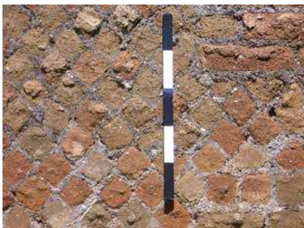
Figure 11.3c: Horrea, via degli Aurighi (III.ii.6). Coarse reticulate of interior face (photo: Janet DeLaine).
