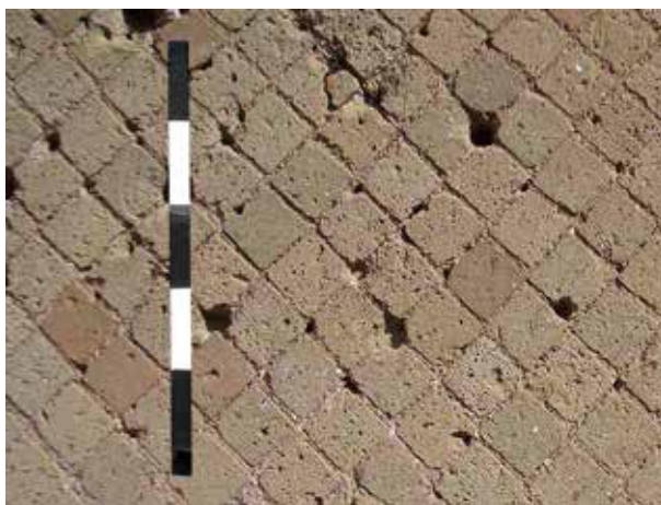
Figure 11.3b: Horrea, via degli Aurighi (III.ii.6). Fine reticulate of façade (photo: Janet DeLaine).
