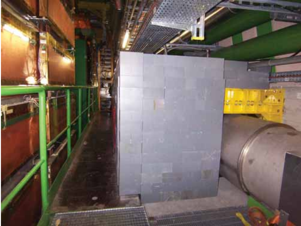
Figure 4.2: Additional shielding installed behind M5 during LS1.
