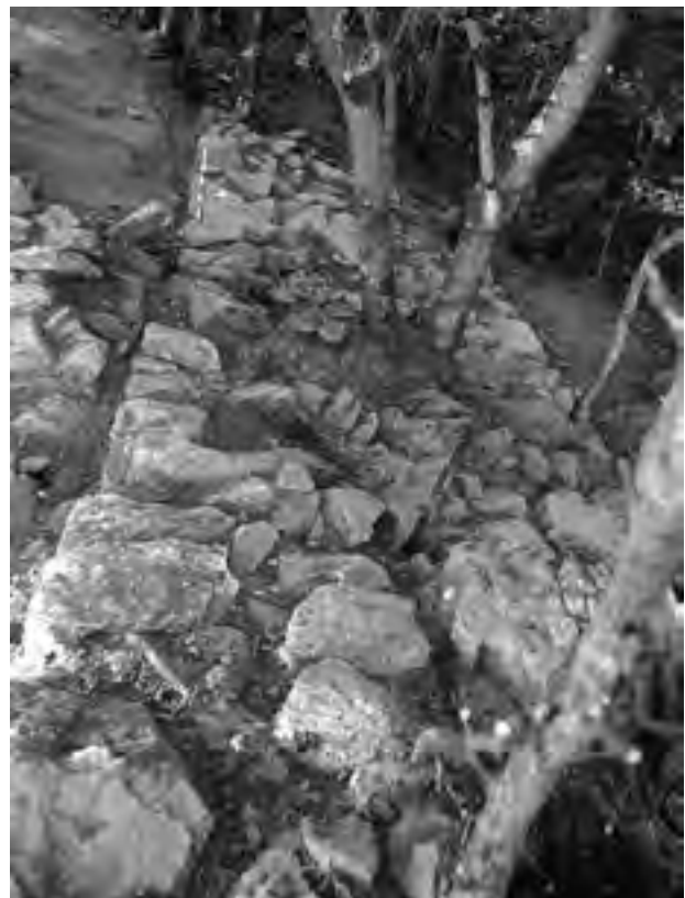
FIGURE 4. Detail of the rampart of Puig Castell), after Guàrdia 2015, 55, fig. 4.
