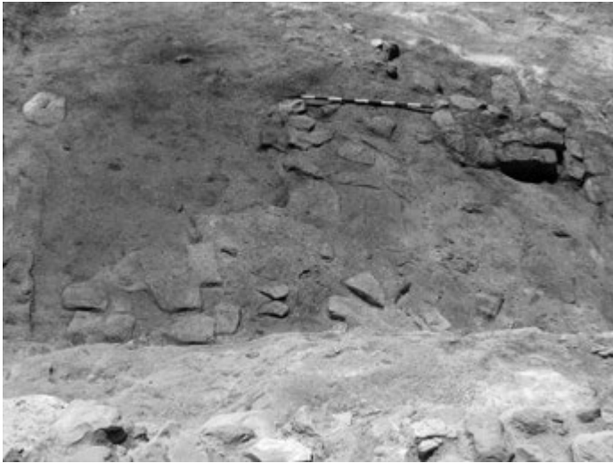
Fig. 4. Mudbrick destruction structures at Sebes, 5th century BC (Flix, Tarragona) (by M. C. Belarte).
